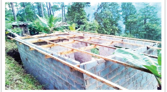
New home under construction
